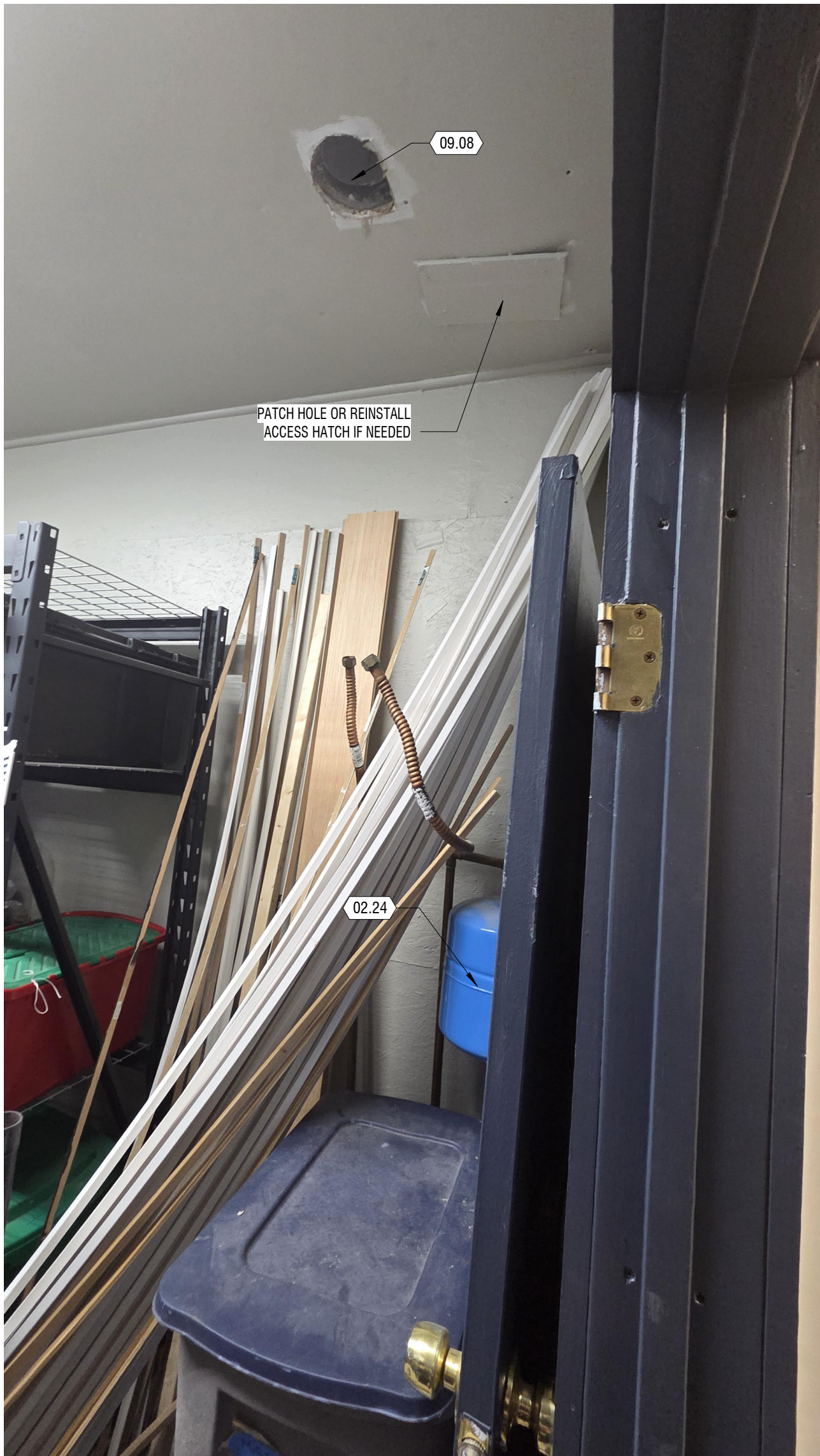
A2 IMAGE - DEMO - OLD WATER HEATER
