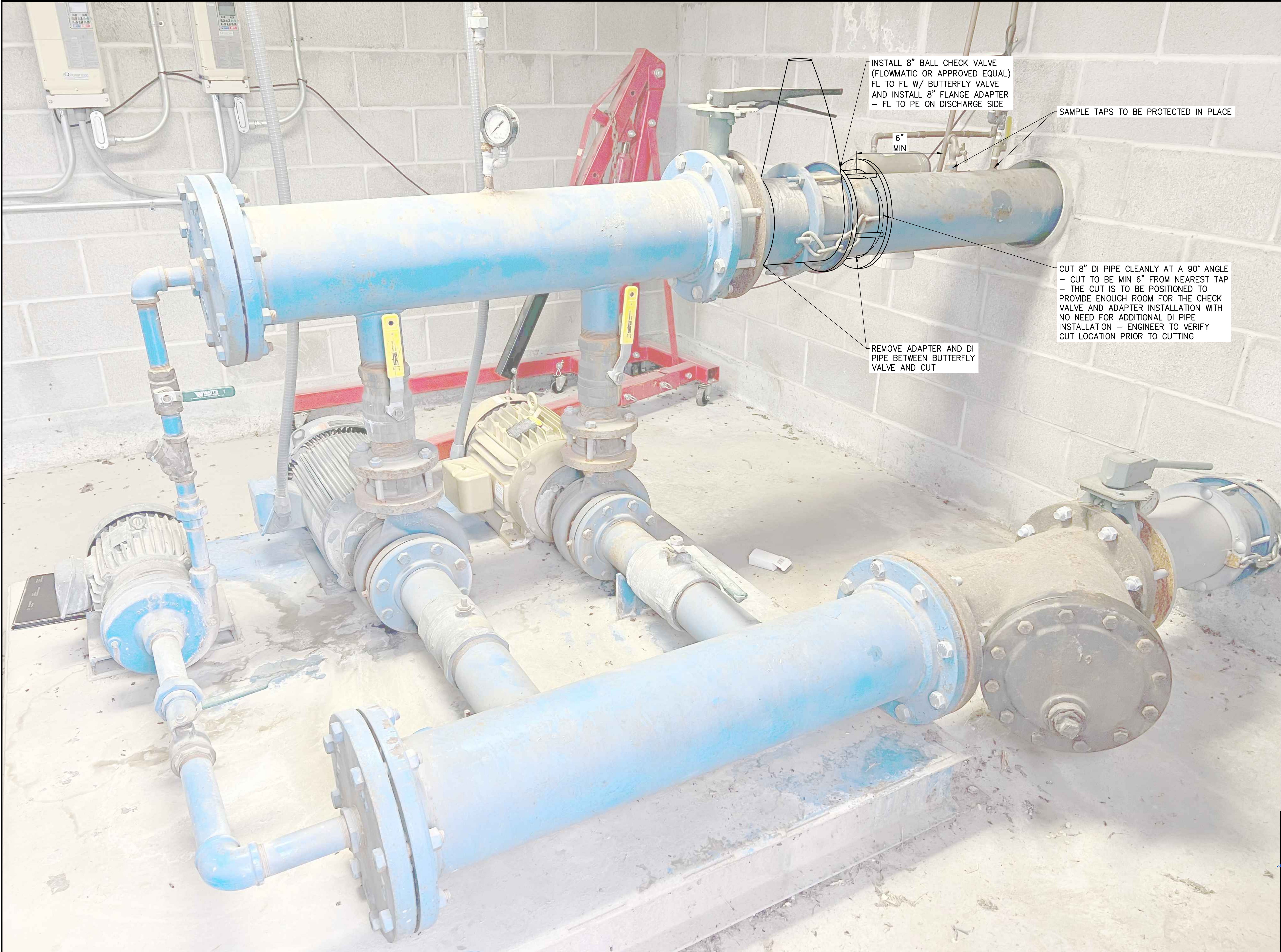
A DETAIL - EXISTING PUMP HOUSE REPLUMBING ~ NOT TO SCALE
