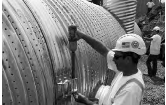
Tightening bolts on a corrugated band.
