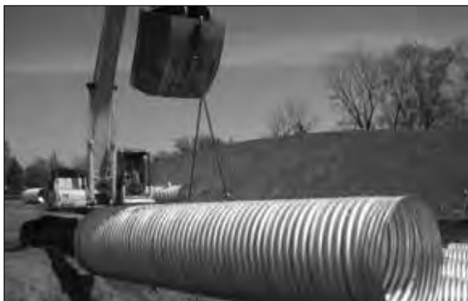
Lifting CMP utilizing factory attached lifting lugs
