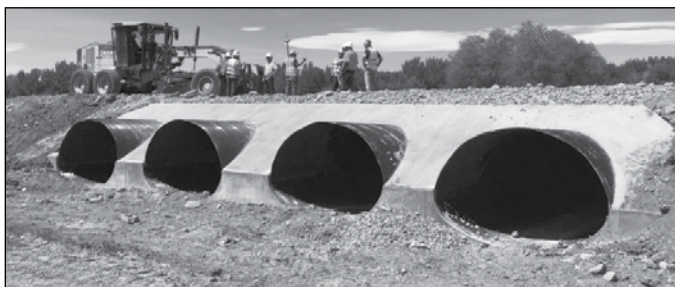
Examples of Multi-Barrel CMP Culverts
