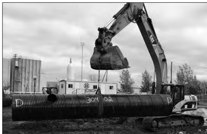
Lifting polymer-coated CMP with nylon straps
