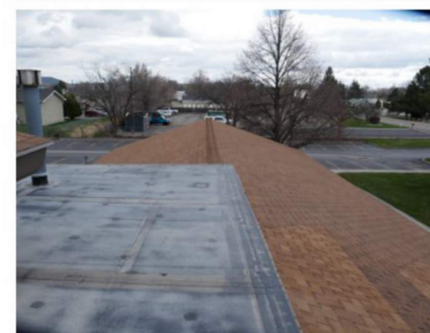
Remove existing wall flashings, install new after installation of new shingles.
