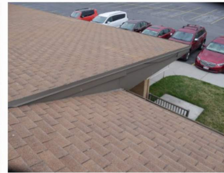
New membrane at low slope area.
