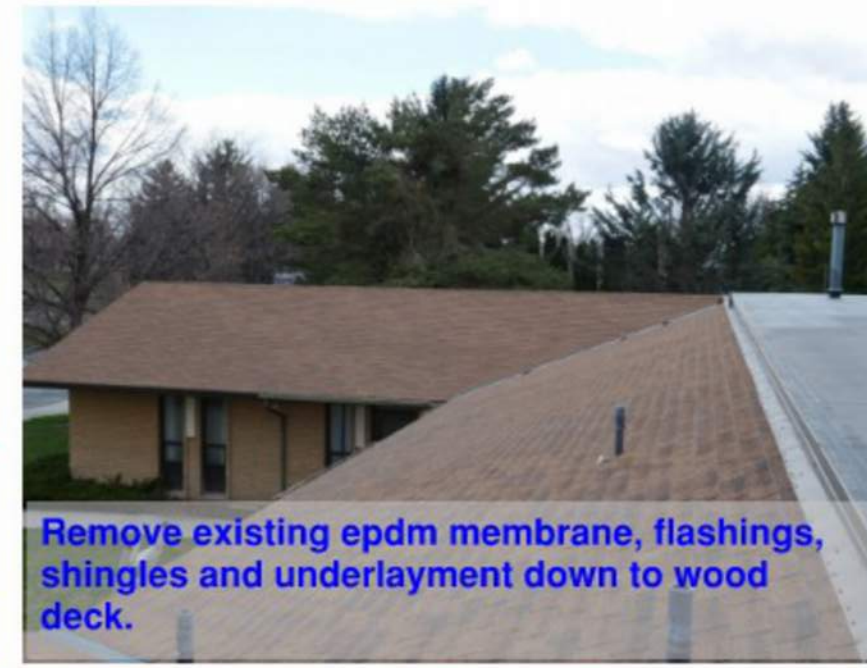
Remove existing epdm membrane to roof deck. Examine deck in presence of architect. Install new 1/2" densdeck and 80ml membrane.
