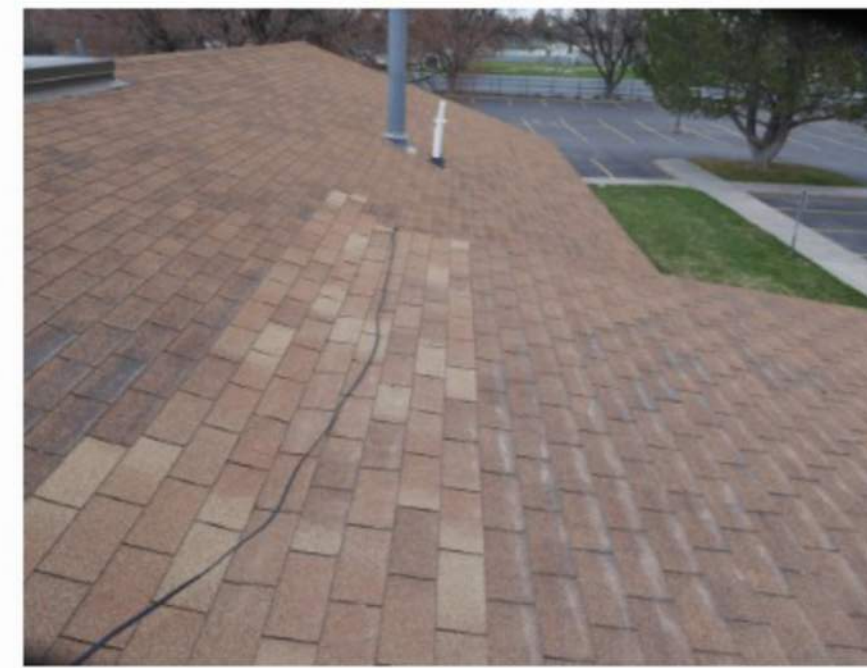
Install pitch pocket where conduit penetrates roof. Remove flashings, install new after installation of new membrane.
