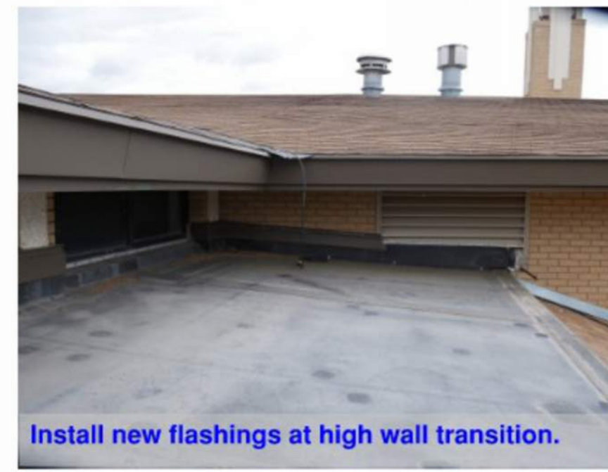
Remove existing flashings and counterflashings. Install new after installation of new roofing. Match fascia color.
