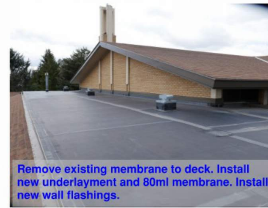
Remove existing membrane, shingles, flashings and underlayment. Install 1/2" densdeck over flat roof area and low slope area. Install new 80ml roofing membrane. Color of membrane to match new composition shingles.
