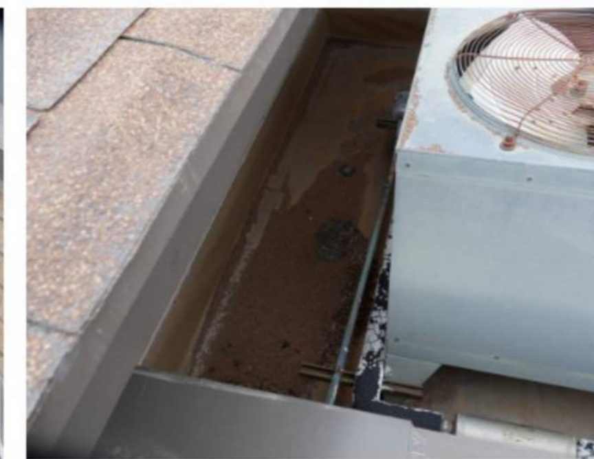
Remove edge metal, membrane, flashings and shingles prior to installation of new materials.
