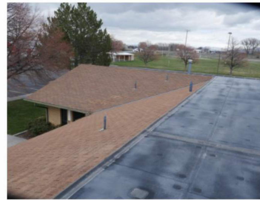
Remove existing shingles, underlayment, valley metals, install new secondary underlayment over entire roof deck. Install new valley metal, composition shingles, new drip edge, etc.
