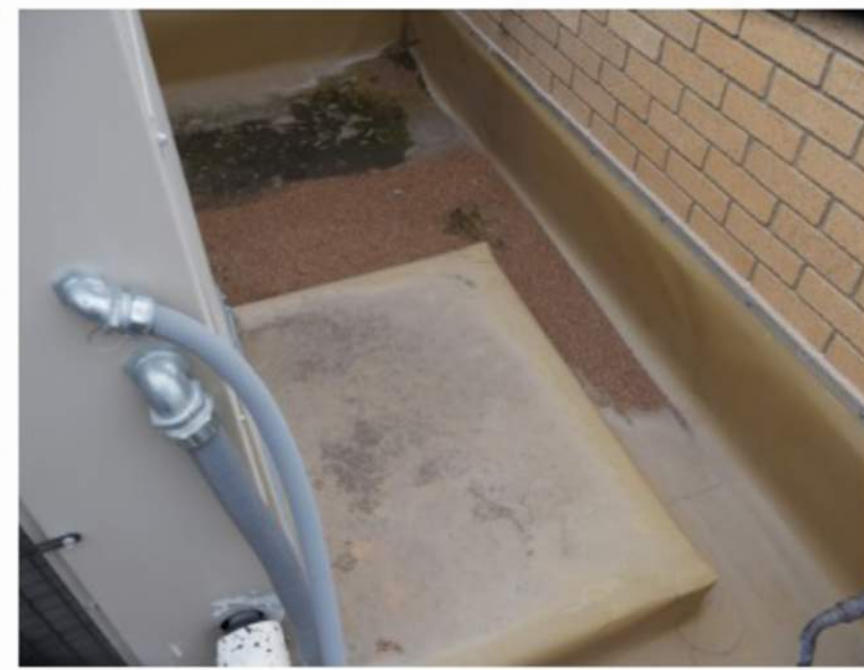
Replace insulation with new. Coat with armaflex paint and cover with new continuous metal.
