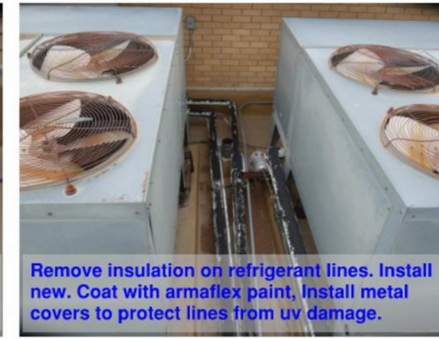
Remove insulation on refrigerant lines. Install new. Coat with armaflex paint, install metal covers to protect lines from uv damage.
