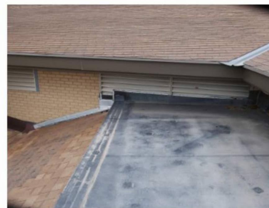
Remove flashings at steeple. Install new to match existing fascia metal. Remove existing shingles and underlayment to roof deck. Install new secondary underlayment over entire roof deck. Install new composition shingles.
