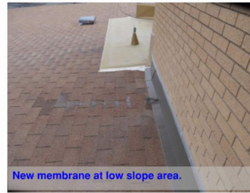
Install 1' x 2' piece of sacrificial membrane where condensate drips onto roof.
