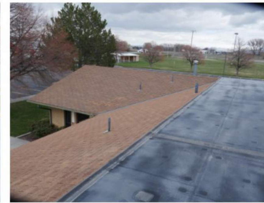
Remove existing shingles, underlayment, valley metals, install new secondary underlayment over entire roof deck. Install new valley metal, composition shingles, new drip edge, etc.
