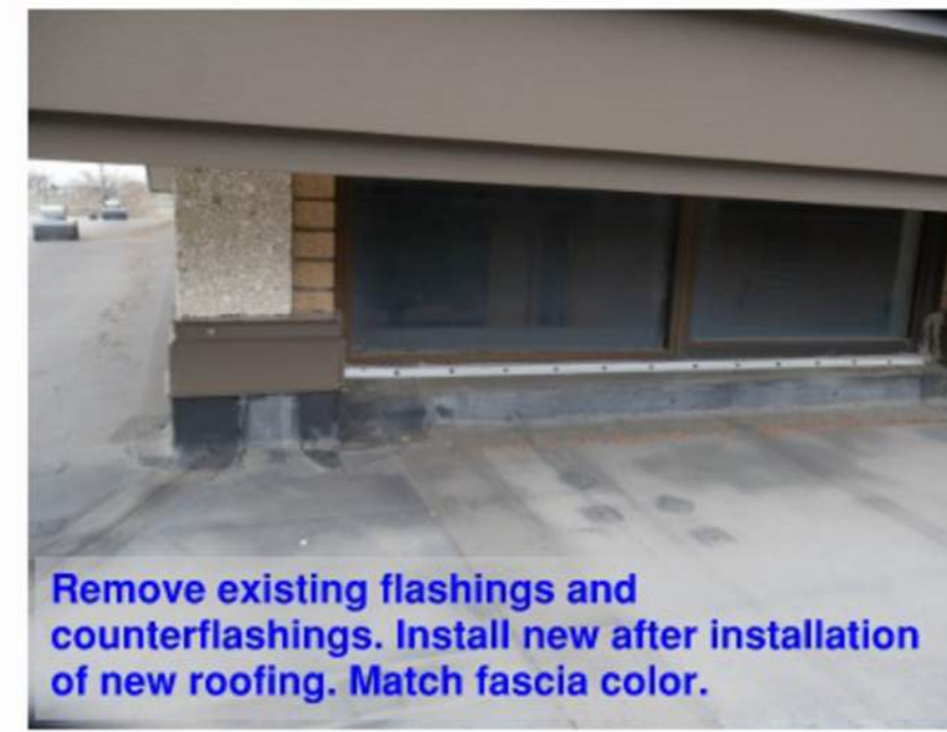
Remove existing flashings and counterflashings. Install new after installation of new roofing. Match fascia color.
