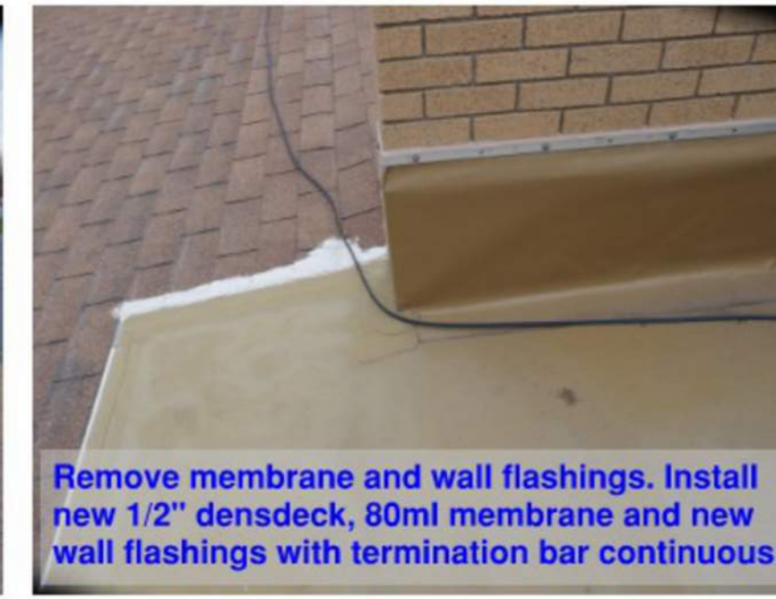
Remove edge metal, membrane, flashings and shingles prior to installation of new materials.
