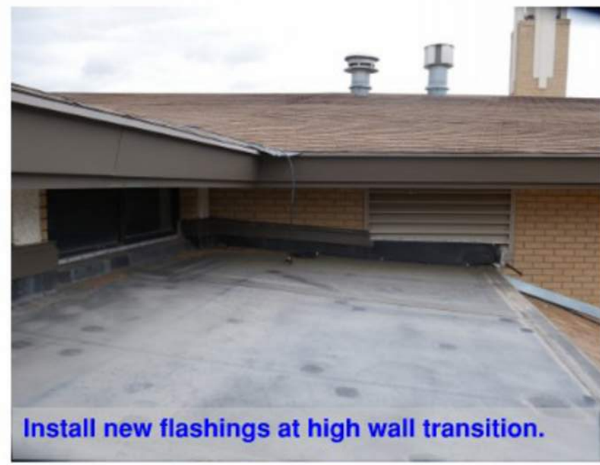
Remove existing flashings and counterflashings. Install new after installation of new roofing. Match fascia color.
