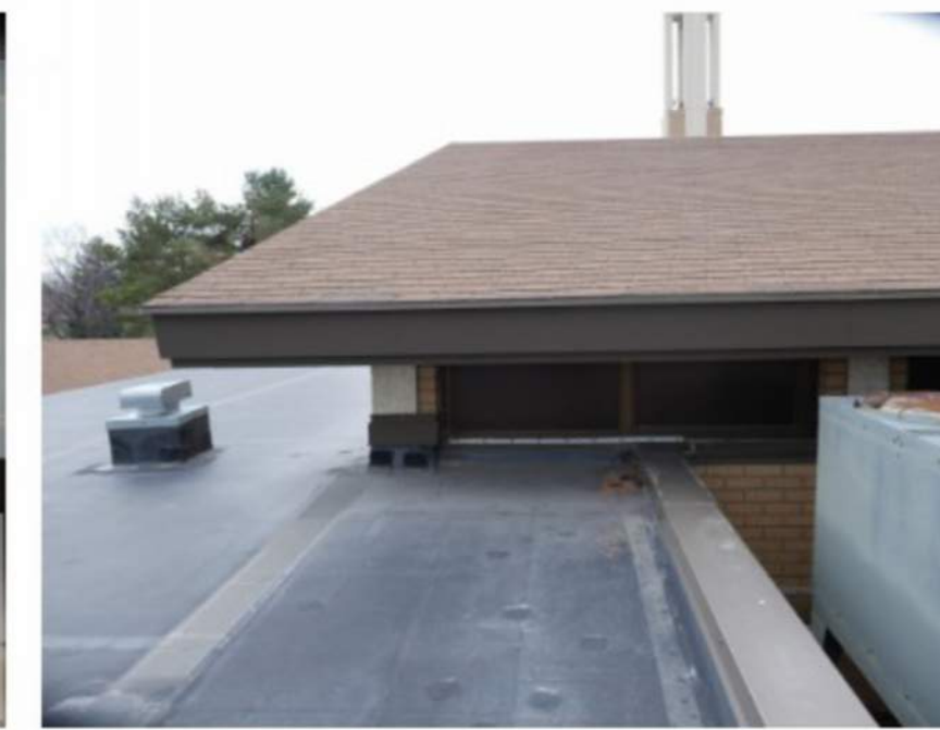
Remove insulation on refrigerant lines. Install new. Coat with armaflex paint, install metal covers to protect lines from uv damage.
