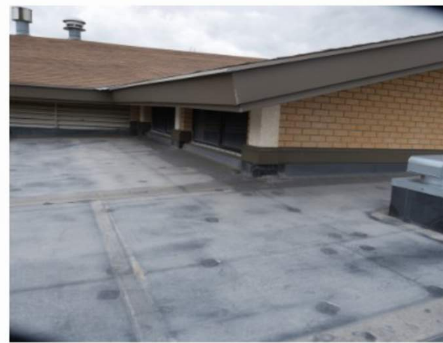
Remove flashings at steeple. Install new to match existing fascia metal. Remove existing shingles and underlayment to roof deck. Install new secondary underlayment over entire roof deck. Install new composition shingles.
