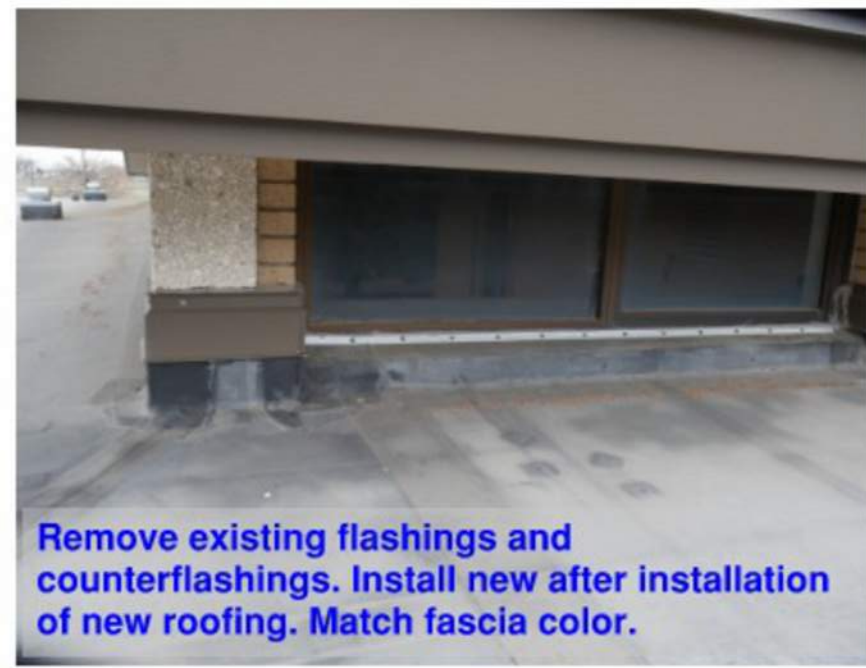
Remove existing flashings and counterflashings. Install new after installation of new roofing. Match fascia color.
