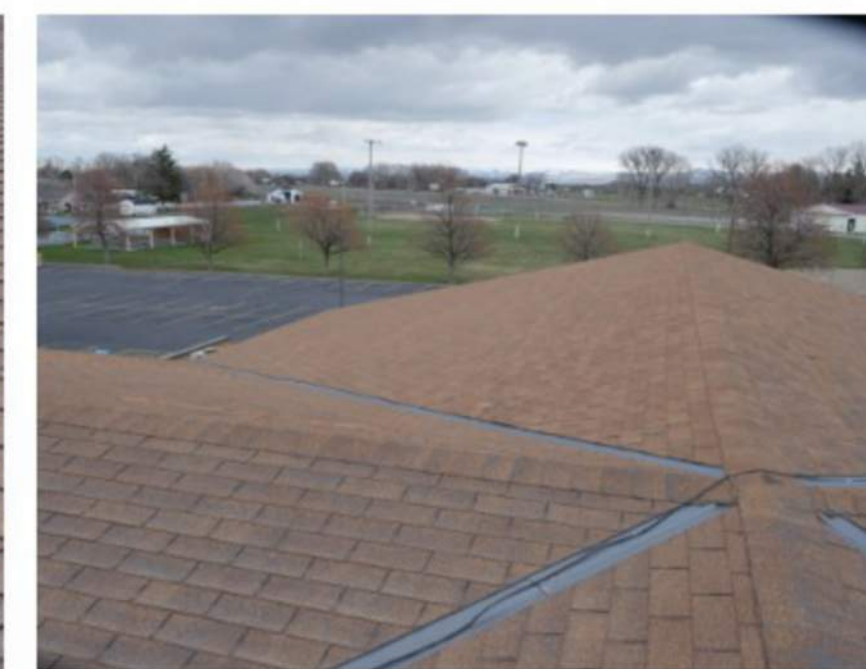
Remove existing wall flashings, install new after installation of new shingles.
