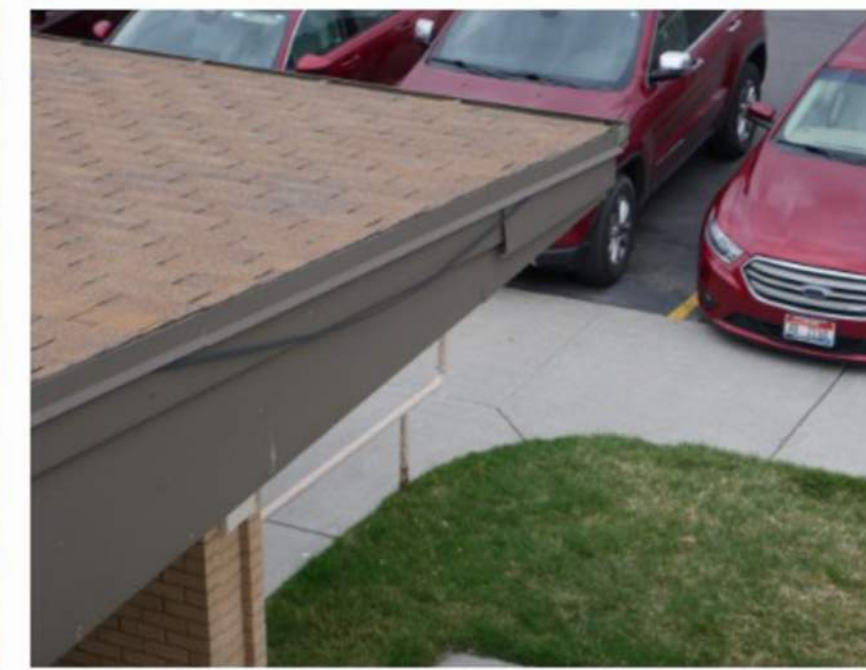
Install 1' x 2' piece of sacrificial membrane where condensate drips onto roof.
