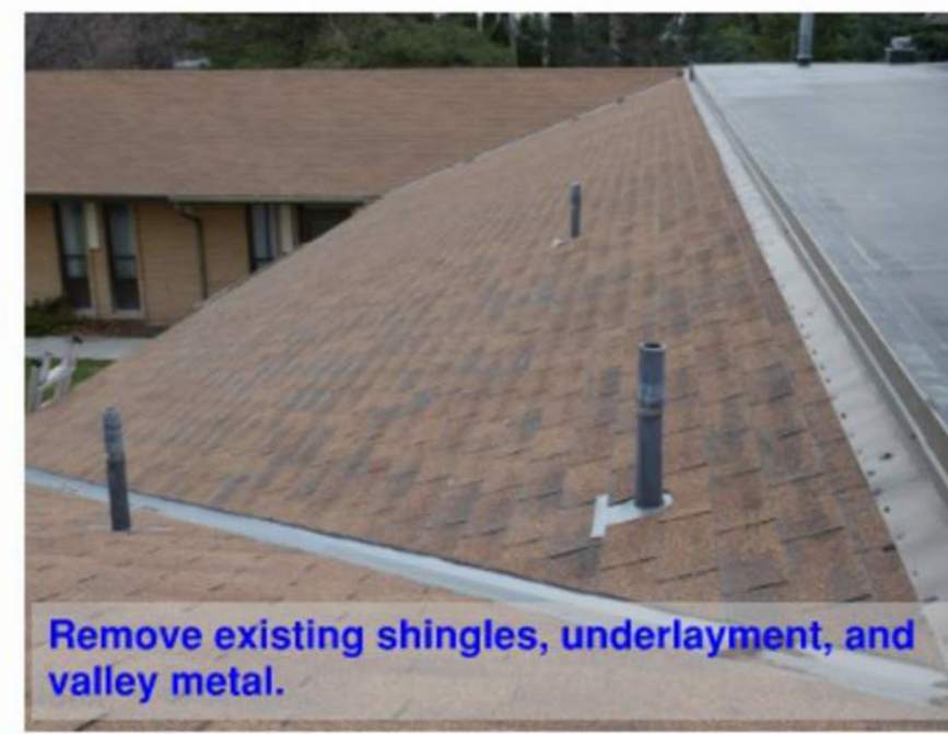
Remove existing epdm membrane, flashings, shingles and underlayment down to wood deck.
