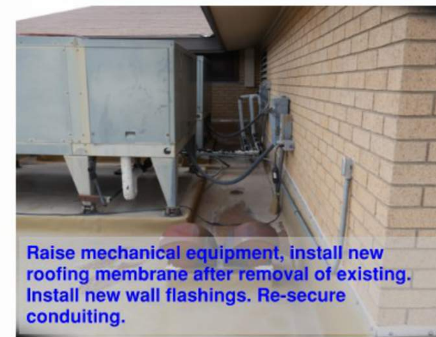
Remove edge metal, membrane, flashings and shingles prior to installation of new materials.
