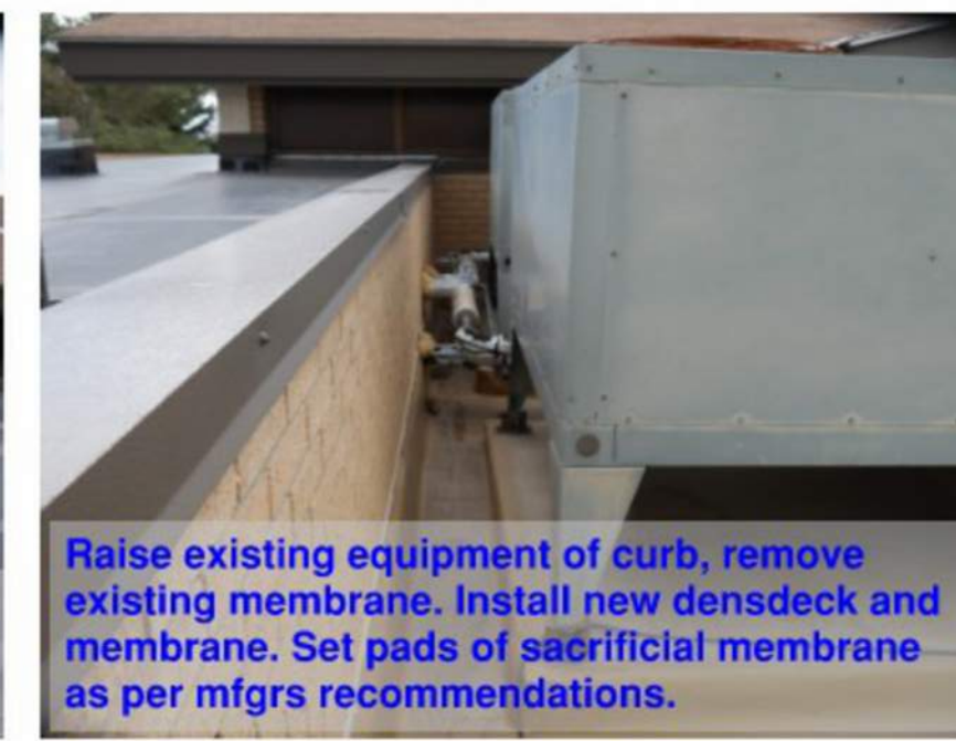
Remove membrane and wall flashings. Install new 1/2" densdeck, 80ml membrane and new wall flashings with termination bar continuous.
