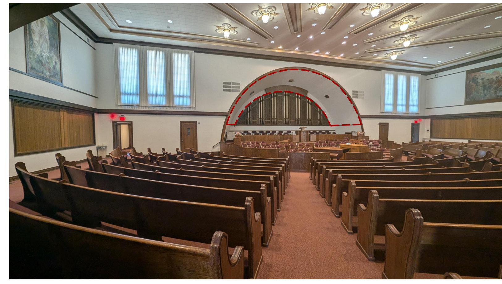
C3 ASBESTOS AT ROSTRUM
