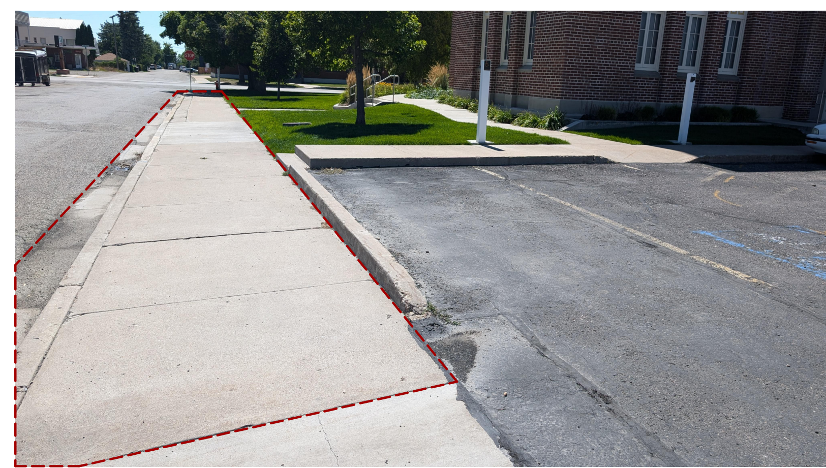
A3 EAST SIDEWALK & CURB REPLACEMENT
