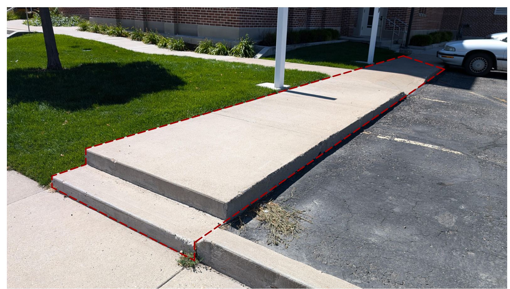
A1 ADA RAMP REPLACEMENT
