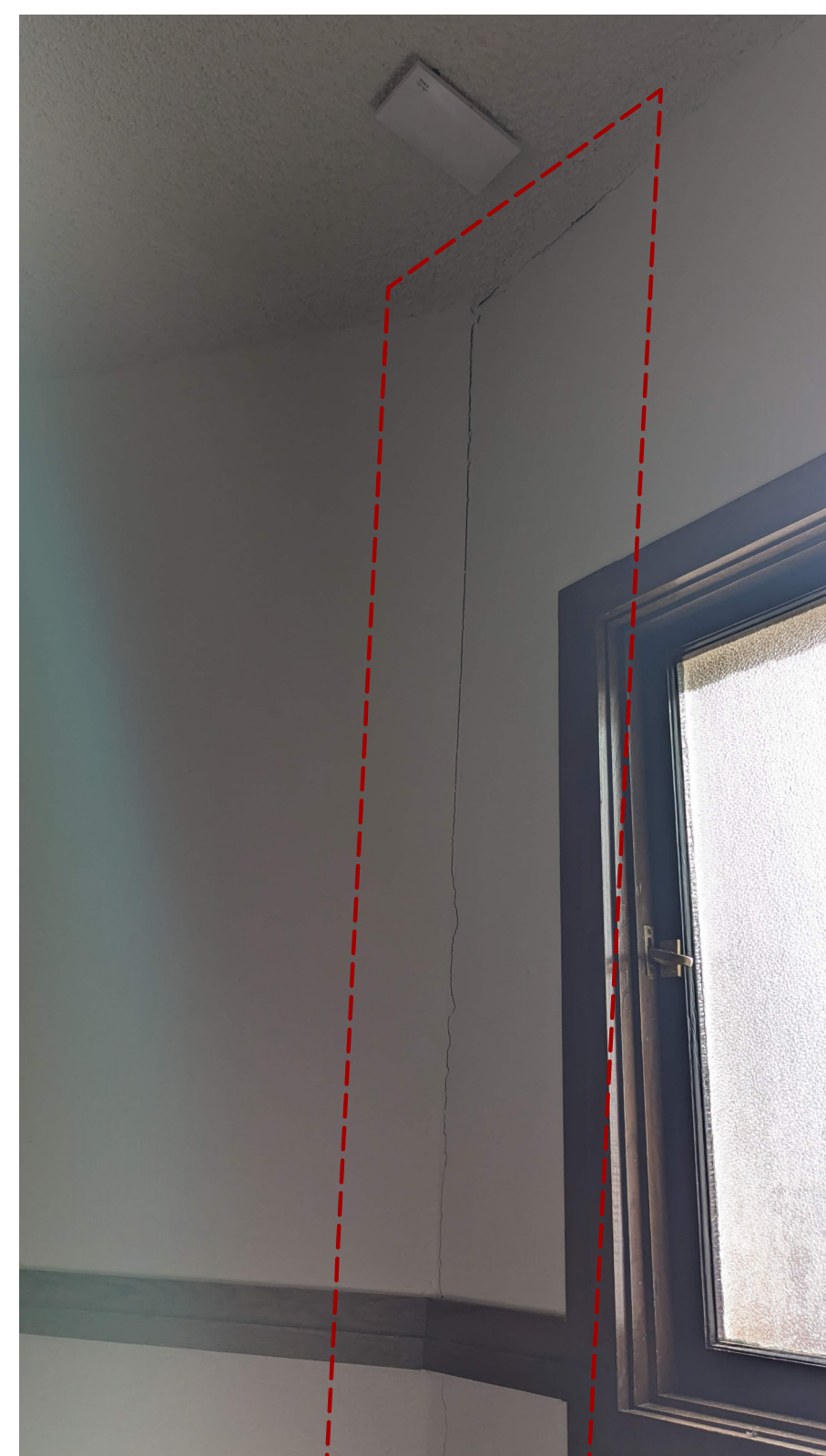
A2 CRACK AT UPPER STAIR WALL
