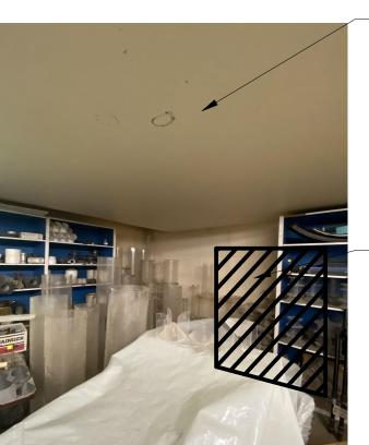
REMOVE EXISTING GYP.BD CEILING, EXPOSE TRUSSES. COORDINATE REMOVAL W/ USU FACILITIES-ABATE ASBESTOS AS REQUIRED.
